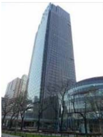
No.5 – Development site for Tokyo Midtown (Above photograph was taken after its completion)
